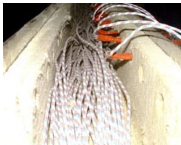
Arrange the wiring of the resistances in a homogeneous way in the tunnel created by the insulators
